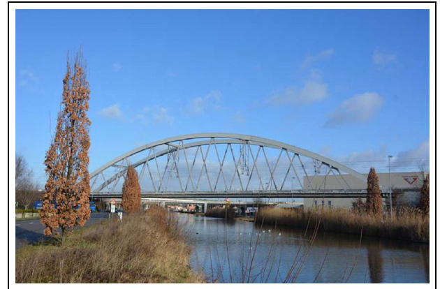
Figure 8. KW51 railway bridge.
